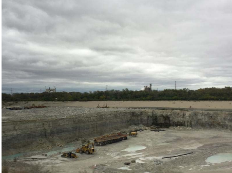
Stage 2 of the McCook Reservoir. Mining equipment ready for action.
