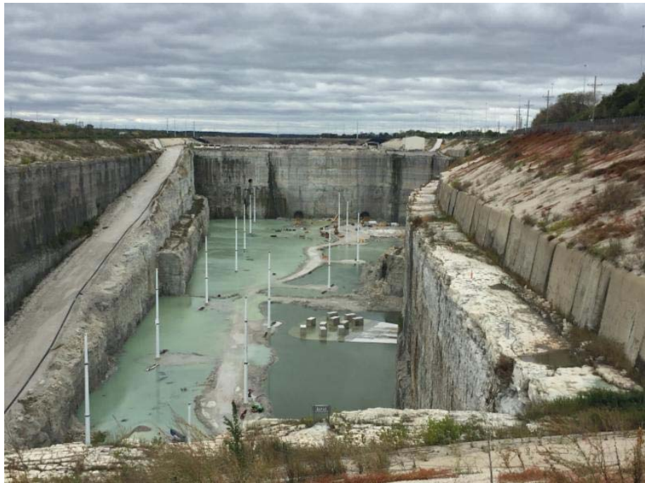
Stage 1 of the McCook Reservoir. The white masts in the center are 150 feet high and will be used to anchor aerators to reduce odor.
