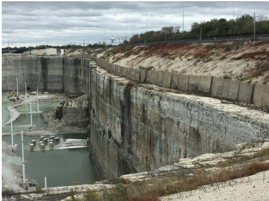
Stage 1 of the McCook Reservoir. The blocks on the floor of the reservoir will help reduce erosion from the inflow of stormwater.
