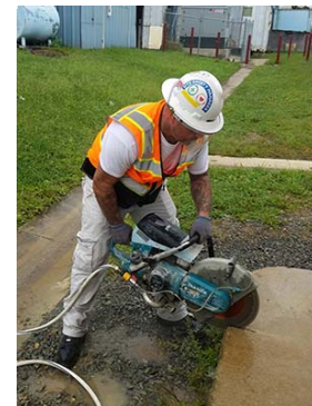
Applying water to a saw blade when cutting materials that contain crystalline silica - such as stone, rock, concrete, brick, and block - substantially reduces the amount of dust created during these operations.
